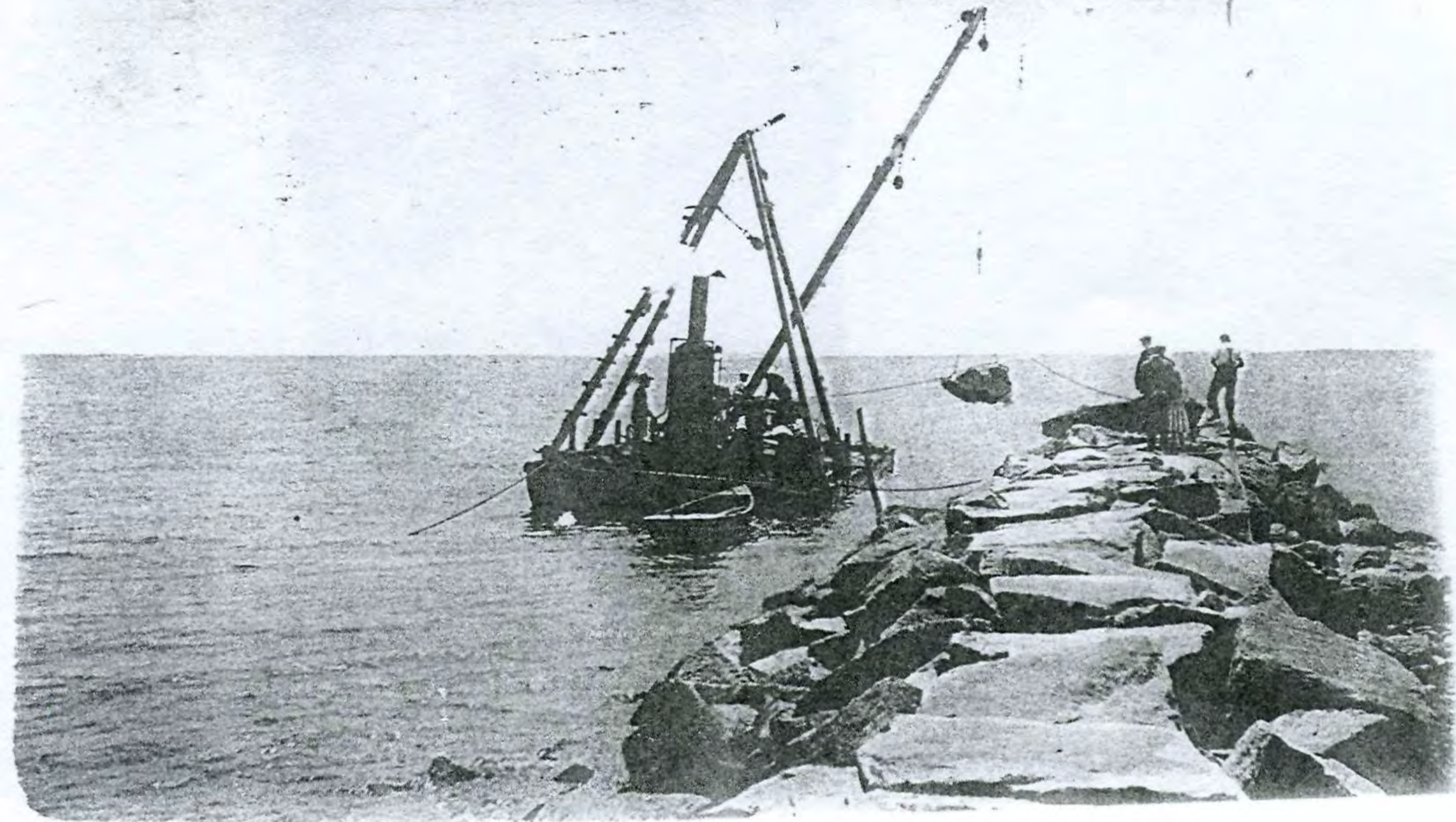
Building the Breakwater, Belmont Beach, West Harwich, Mass.
