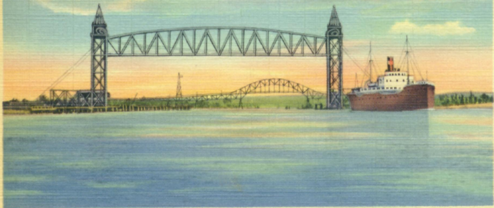
151 RAILROAD AND BOURNE BRIDGES OVER THE CAPE COD CANAL
